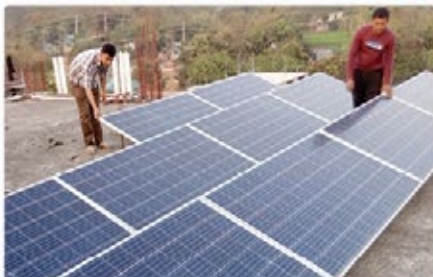
New solar panels keep security lights and CCTV cameras operating 24 hours a day
